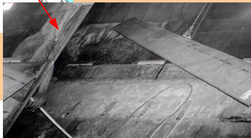
Stainless Steel Cricket Being Added To Existing Wet-Bottom Ash Hopper
